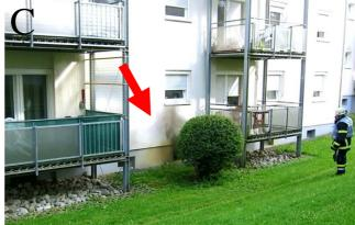
One window in the basement showed smoke coming out in a pulsing way, indicating that there is a moderat fire in the basement which is underventilated and probably some "plastic material" is involved. Several windows have been open in the apartments on Side C.
